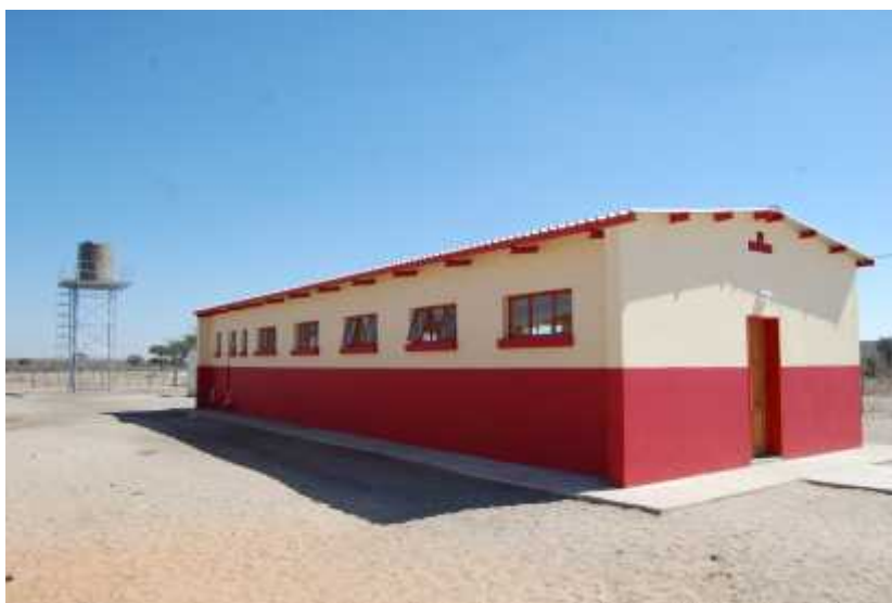
Our dormitory and Eiseb and the newly constructed water tower and tank
