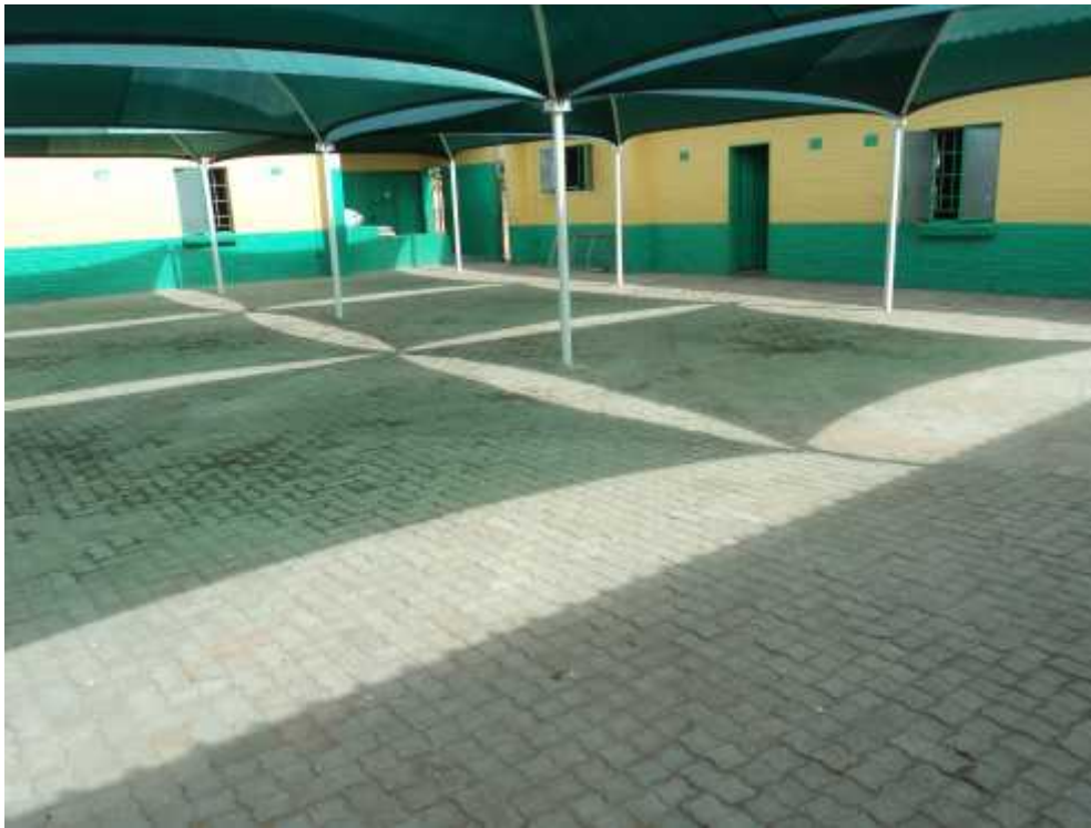
Covered seating after having been block paved.
