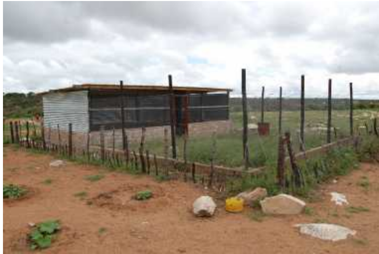
The partially completed chicken run.
