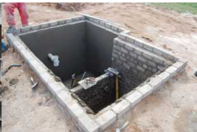
The septic tank under construction
