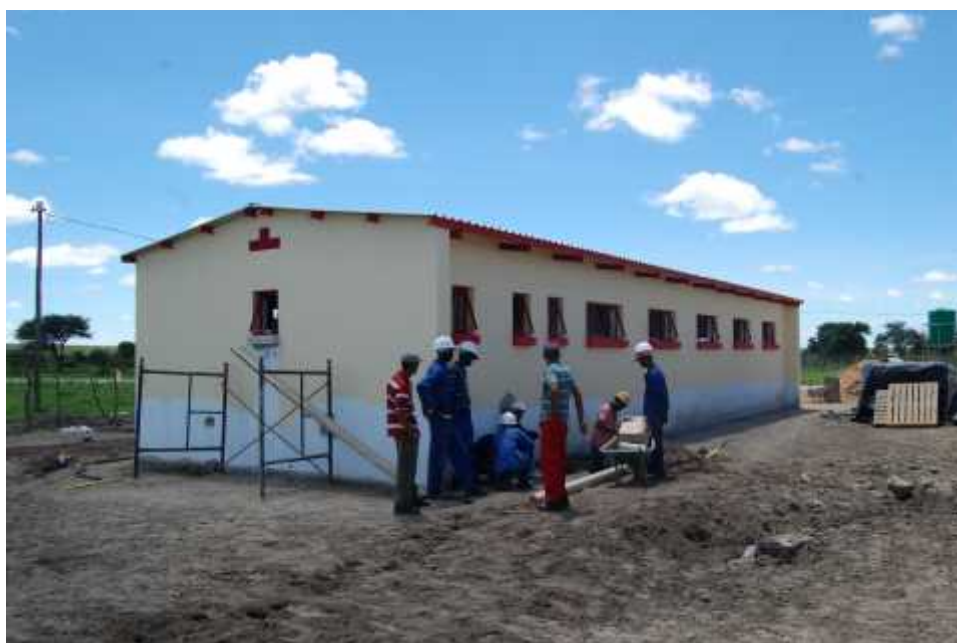
Our dormitory well on the way to completion.
