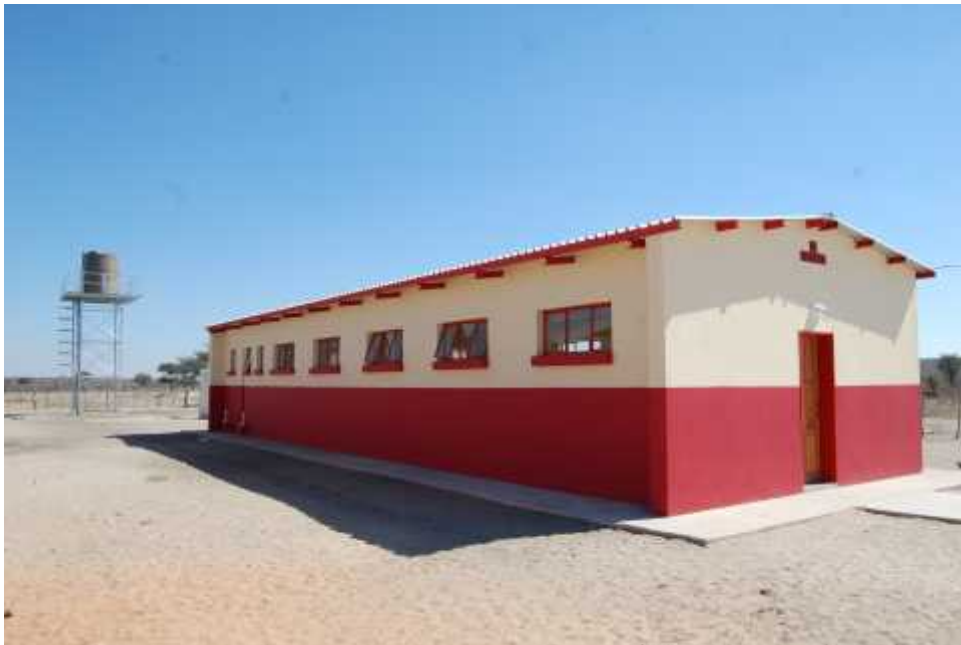
The new dormitory at Eiseb Primary School Hostel
