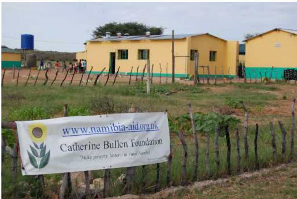
The newly built kitchen at Omuhaturua Primary School Hostel
