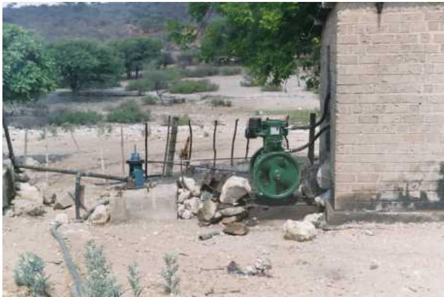
The borehole at Omuhaturua Primary School refurbished to provide fresh water for the school and the village of Otjimanangombe.
