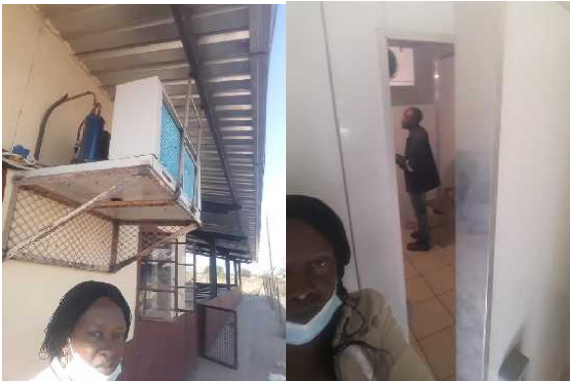
The school secretary, Ngero Tjitunga, underneath one of the air conditioning cooling units and by the door of the new cold room.
