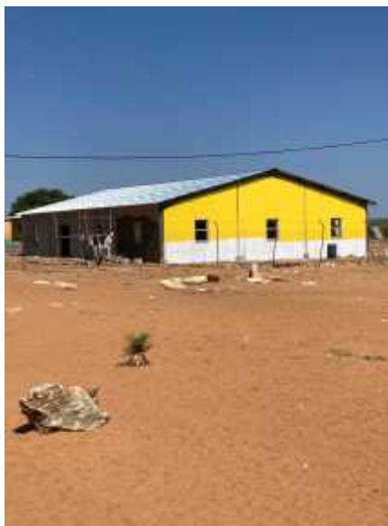
Exterior view, first coat of paint applied
