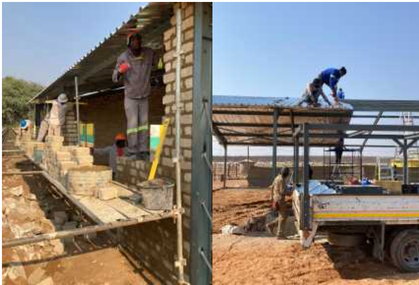
Walls taking shape
