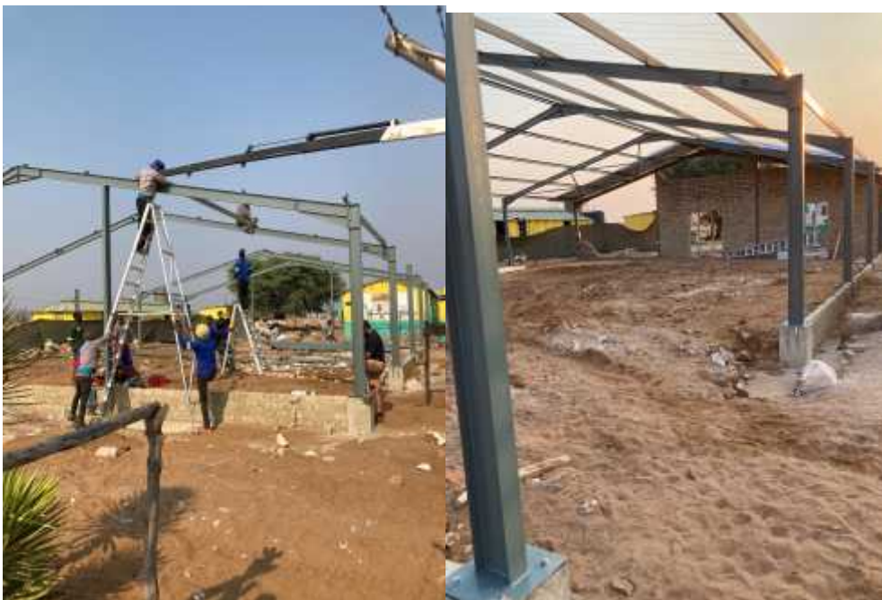
Steel structure starts to take shape
