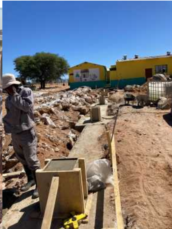
Foundations laid, with the base for the steel uprights.
