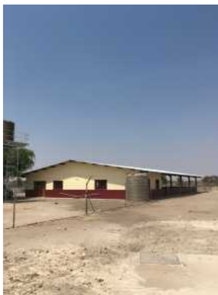
Left: View of the rear of the kitchen with the water tank to harvest the rainwater from the roof. Right: Aluminium cooking pots on the two gas ranges. A big thank you to Kondjeni architects for donating the gas installation including the cylinders, piping and ranges.
